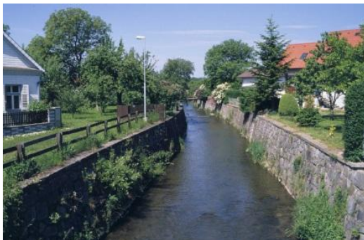
Figure 22: stone pitching tightly packed
