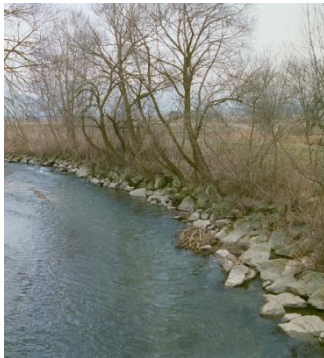
Figure 20: riprap (BOKU, IHG)
